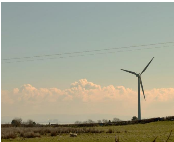
Figure 17: Wind turbine at Peasholme
