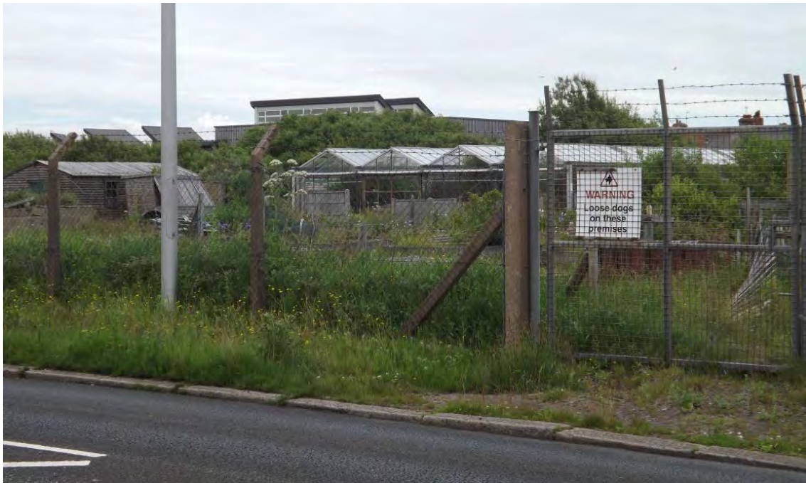
Former garden centre site, Mill Lane, Walney
