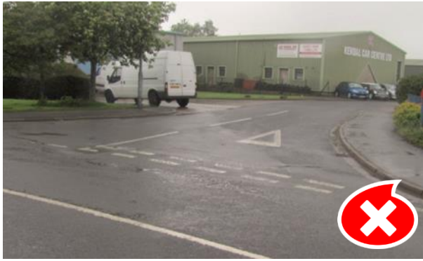
No dropped crossings for pedestrian to use at or near junction
