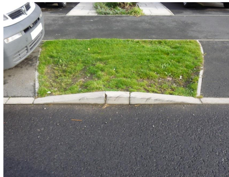
Figure L4: Short landscaped verge causes maintenance issues
