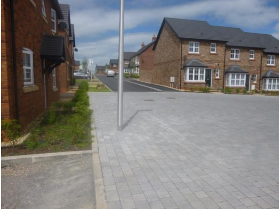
Figure L2: The position of the lighting column within a square puts it at risk of collision with vehicles and pedestrians
