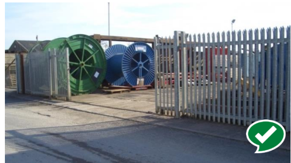
Perimeter gate which opens in parallel to the carriageway and within the site boundary.
