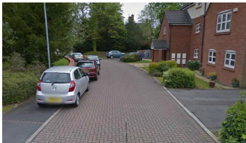
Figure P4: Parking on the footway
