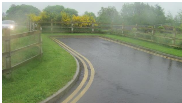
Turning facility treated with yellow line markings
