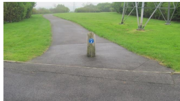
Concrete bollard with shared facility signage
