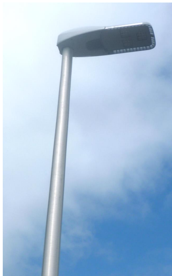
Figure L1: LED lantern used within residential development in Cumbria
