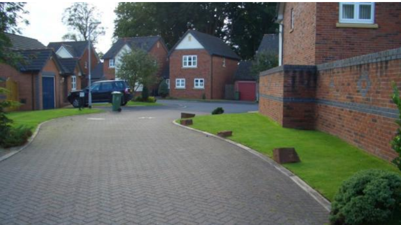
Figure P3: Retrospectively installed makeshift bollards
