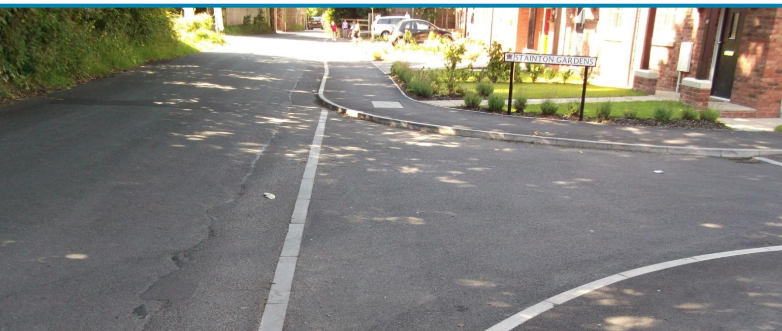
Figure SM3 (below): Flush kerb used as an alternative to a painted give-way marking
