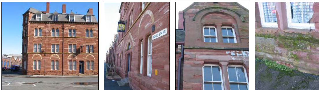
The refurbished Devonshire Public House (middle and far left). The maintenance and repair of surrounding parts of the building can be seen middle and far right.
