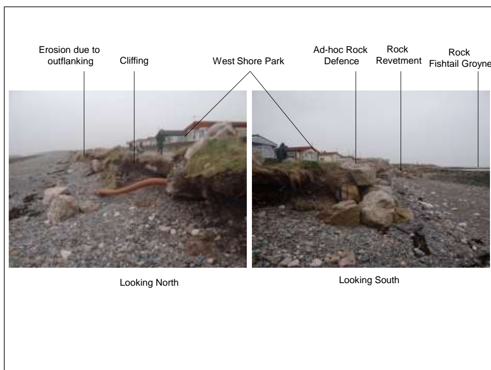
Figure 1 – Erosion at West Shore Park
