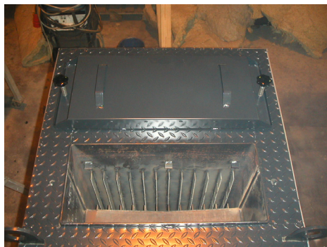
1. Open the sweeping hatches located on the top of the boiler.
