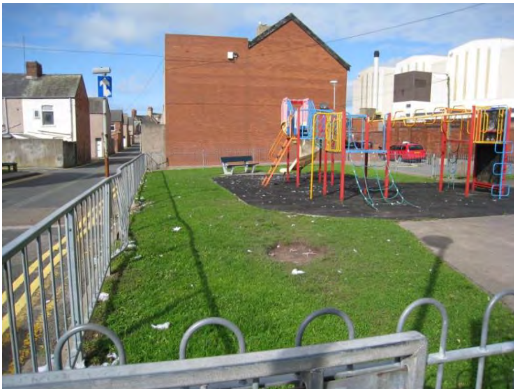
Below: Poor surveillance and lighting at Stanley Road playground, Barrow
