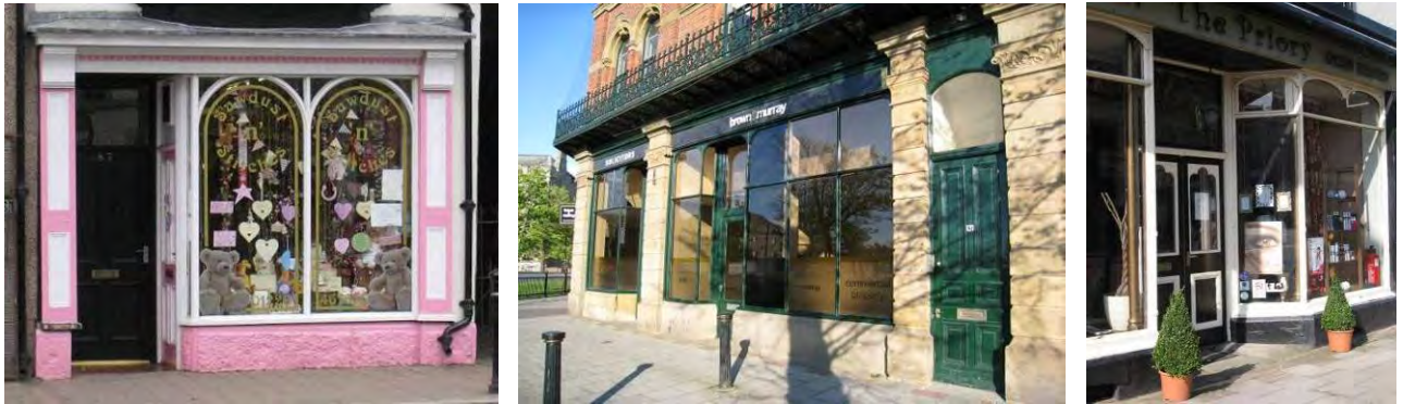
Left: A restored mid Victorian styled shopfront with arched headed windows at Dalton-in-Furness; Centre: An original mid to late Victorian shopfront of c1873 at Ramsden Square, Barrow. Right: 87 Duke Street c1868 which may have had its mullions removed
