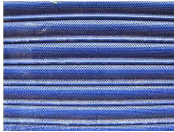
Painted perforated lath type steel roller shutter
