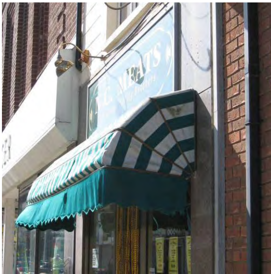
Plastic partly retractable 'Dutch Blind'
