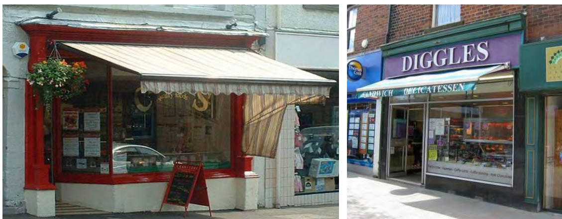
These modern retractable blinds are often suitable modern alternatives if carefully positioned. The original blind box is still in place at Diggles on the right
