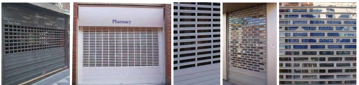
'Punched' 'stamped' or 'cut' type shutter, available in aluminium, steel or plastic and 'Punched' type shutter with transparent polycarbonate vision panels, normally in aluminium
