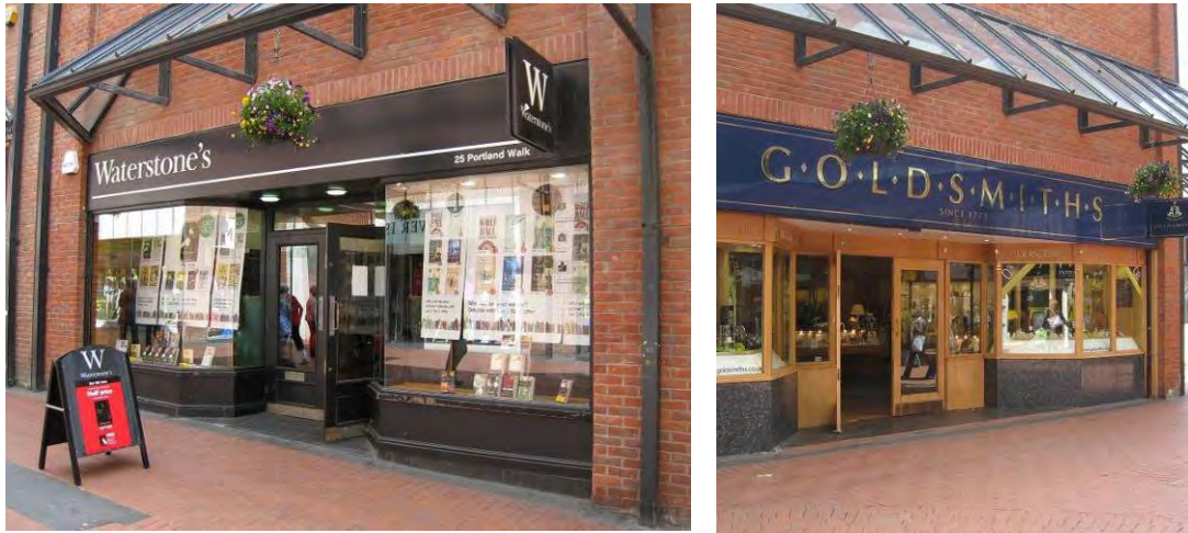
Examples of modern, attractive and well-presented shopfronts in Portland Walk Barrow. Left: A predominantly timber shopfront with modern frameless glazing but with profiling to the timberwork adding dimension, and sitting within the building's brick piers which provide framing, separation and solidity. Right: A more traditional and elaborate timber detailing to this modern shopfront.
