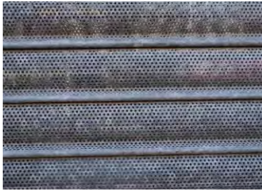
Unpainted perforated lath type steel roller shutter
