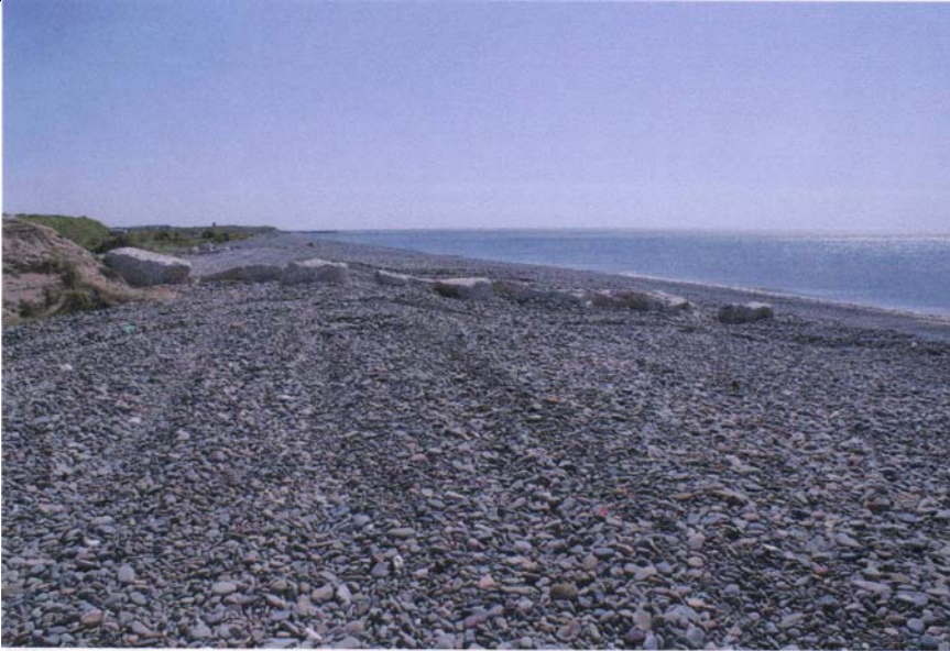
Photo 3: Showing rocks laid out across shingle beach (and vehicle tracks in foreground)
