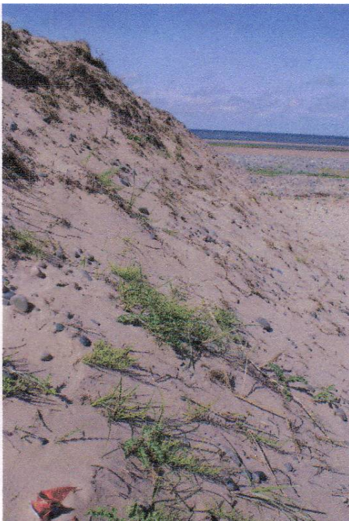
Photo 2: Showing vegetation establishing on surface of re-profiled dune.
